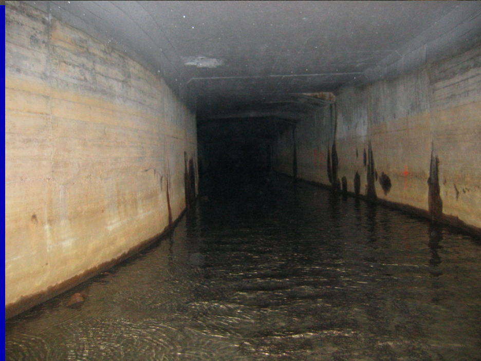
Box Culvert Inspection, February, 2004
